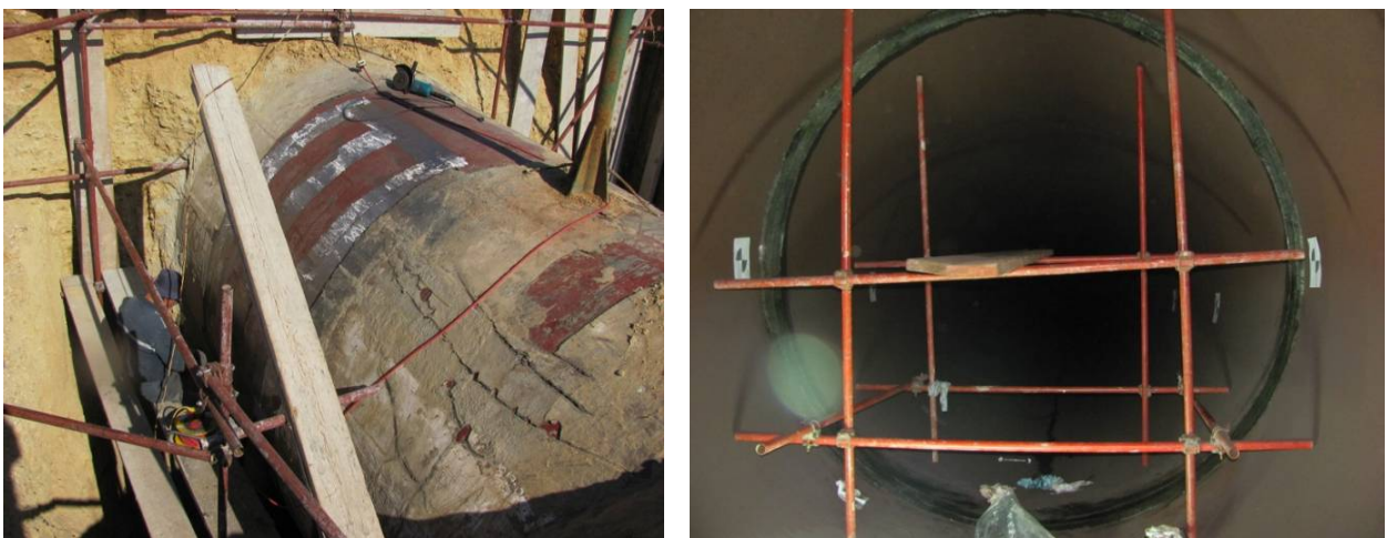
a) Preparation of the external pipeline surface
