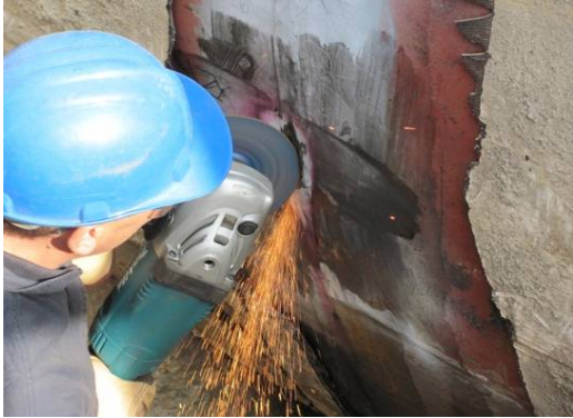
a) Appearance of the repair of a cracked area
