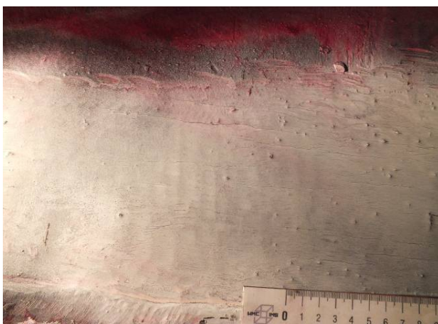
a) Appearance of surface cracks on the surface of parent
