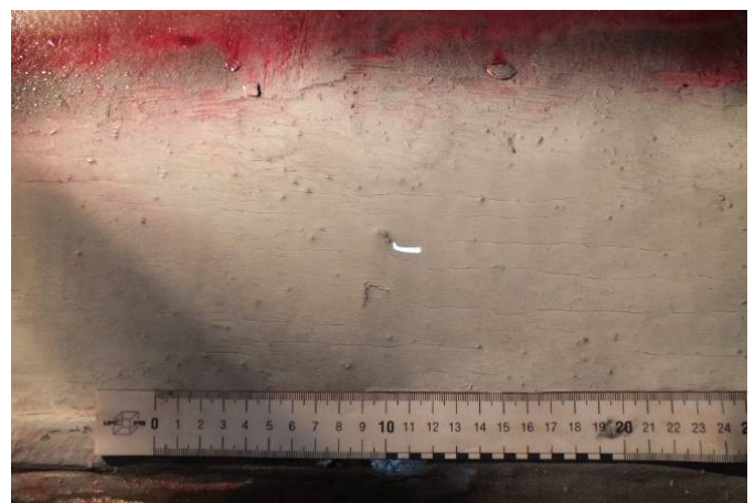
b) Appearance of surface cracks the surface of weld metal material
