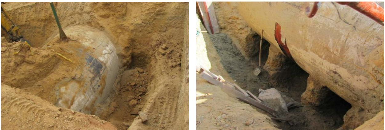
Fig. 2. Appearance of the uncovered pipeline segment
