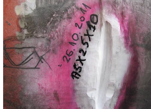
b) An area prepared for surface welding
