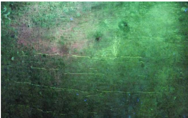
a) Appearance of surface cracks on the surface of parent
