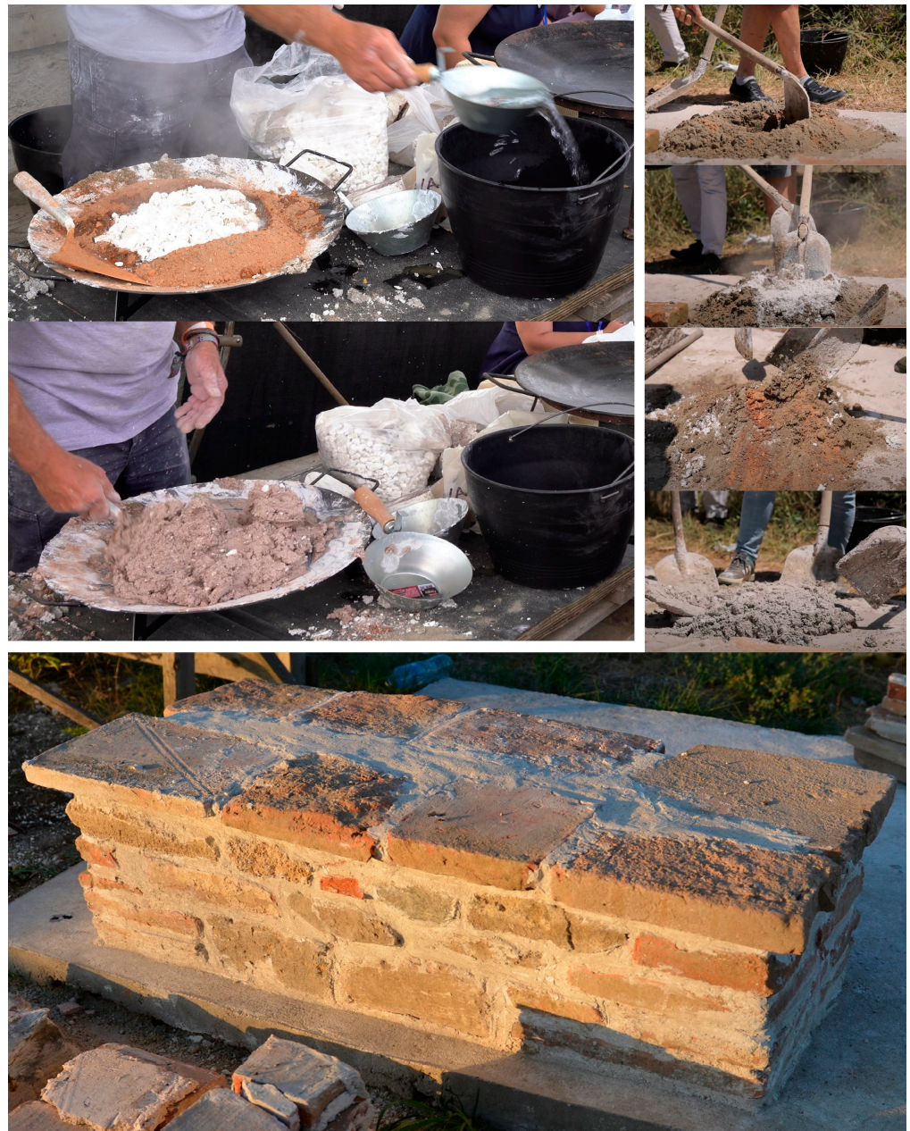
Figure 13. Hot mixing during the MoDeCo2000 workshop. Creating a demonstration mixture ( top left ) and the mixtures for a wall structure using lime mortars, with natural brick as admixture with a photo of the wall 11 days after the building ( top right , and bottom ). Photo documentation of the MoDeCo2000 project.
