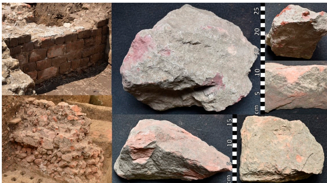
Figure 4. Natural brick in Viminacium legionary fortress, used in the wall of the principium in the form of blocks (top left), and the rampart with natural brick in the form fragments used in the foundations and wall core, as well as fragmented blocks used over ground, along which the later stone phase was erected (bottom left); different fragments of used natural brick collected from the principium site (right). Photo documentation of the MoDeCo2000 project.
