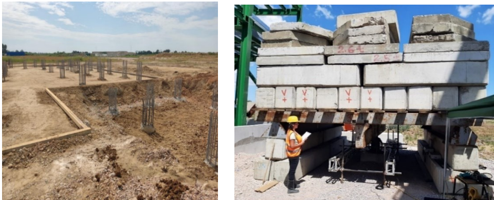
Figure 6. a) Derived piles that have been prepared for testing b) Static load test
