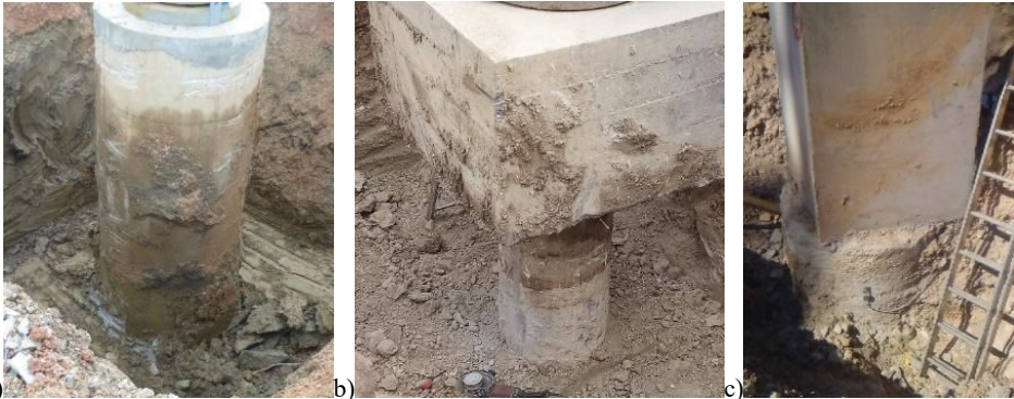
Figure 4. a) adequate preparation, b) partially adequate preparation, c) partially adequate preparation
