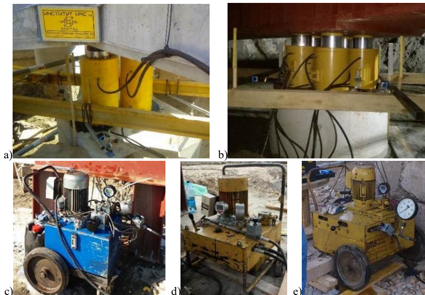
Figure 1. Equipment for testing the load-bearing capacity of piles by Static Load Test (SLT): a) Prva petoletka - IMS press, capacity 2x600t, b) Prva petoletka - IMS press, capacity 6x250t, c) hydraulic system (pump) - Version 1, d) hydraulic system (pump) - version 2, e) hydraulic system (pump) - version 3
