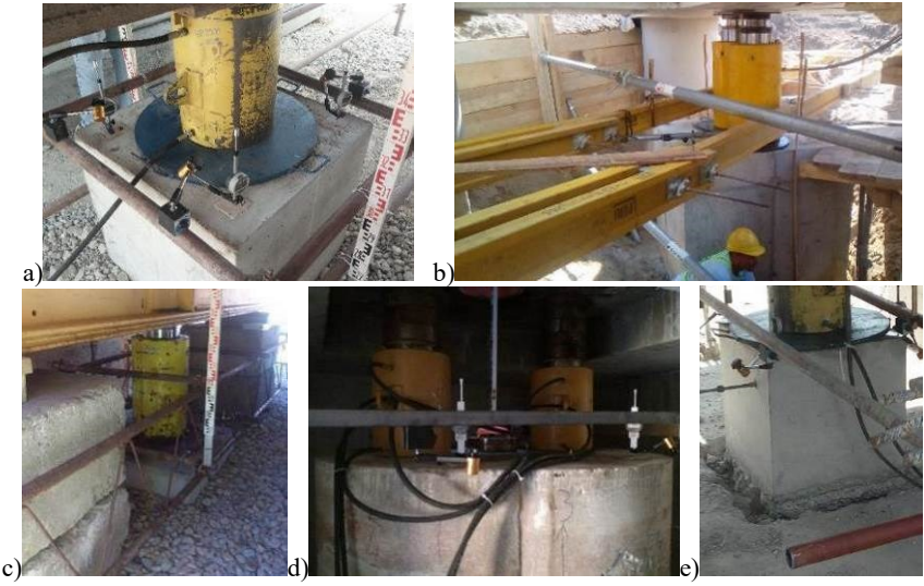
Figure 3. a) comparator positioning, b) reference system formed of wooden beams, c) reference system formed of steel lattice R beams, d) specially designed reference system, e) spacing of the pile cap from the concrete slab
