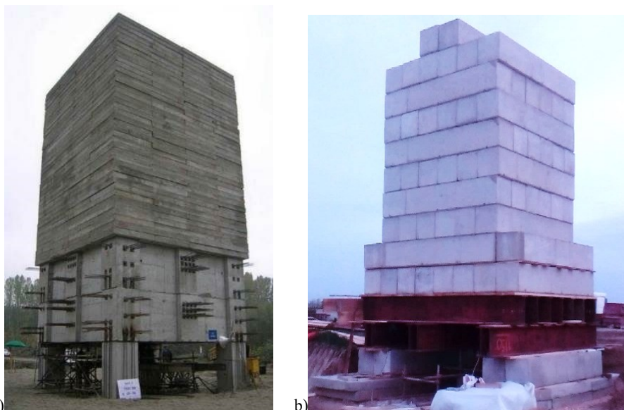
Figure 4. SLT - counterweight: a) The Mihajlo Pupin bridge in Zemun-Borča, Serbia (counterweight formed of reinforced concrete slabs), b) wind farm Malibunar in Serbia (counterweight formed of reinforced concrete blocks)
