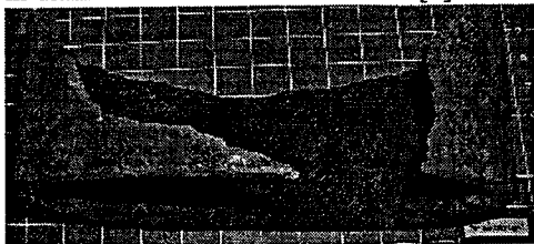
Figure 1 – Heavily corroded gray cast iron pipe
