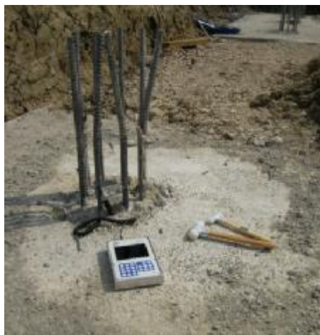
Slika 7: Savremena oprema SIT PRO za ispitivanje šipova u vlasništvu Instituta IMS. Figure 7: The modern SIT PRO pile testing equipment owned by the IMS Institute
