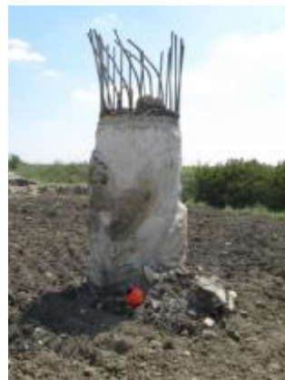
Slika 10: Loš kvalitet betona pri vrhu šipa: a) reflektogram i b) otkriven šip. Figure 10: Poor quality concrete at the pile top: a) reflectogram b) the exposed pile
