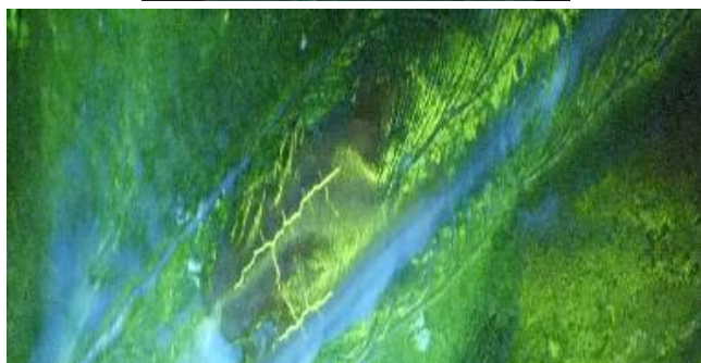
Figure 9. Defects detected in parent material and welded joints of anchor of breeches pipe no.1.
