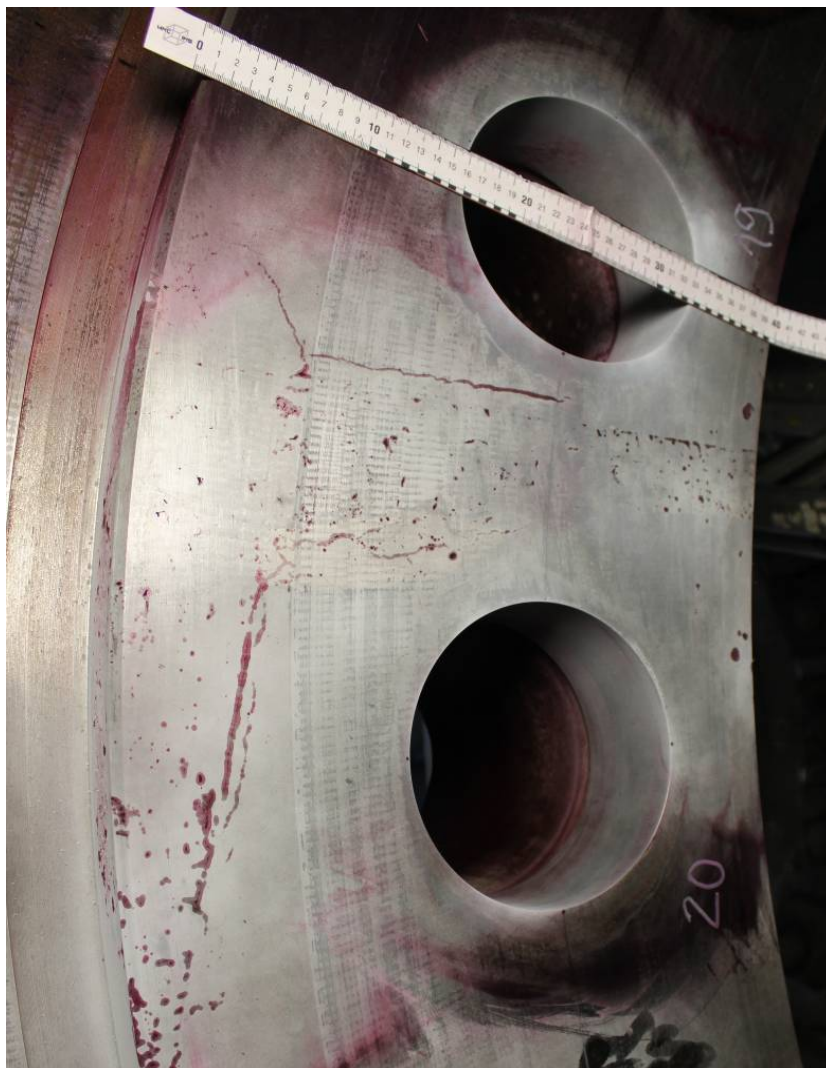
Figure 5. Cracks in the area of the repair weld (between openings for bolts nr. 19 and 20).
