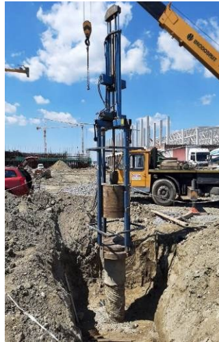
Figure 2. Equipment for in-situ DLT of the pile
