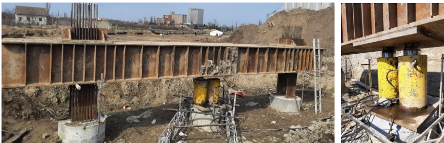
Figure 1. Reaction system consisting of a reaction beam anchored in two piles
