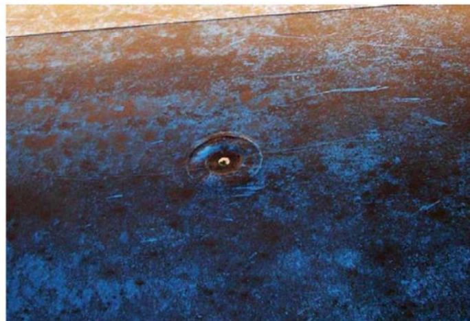
Figure 7. An example of a zinc reference electrode on a ship's hull
