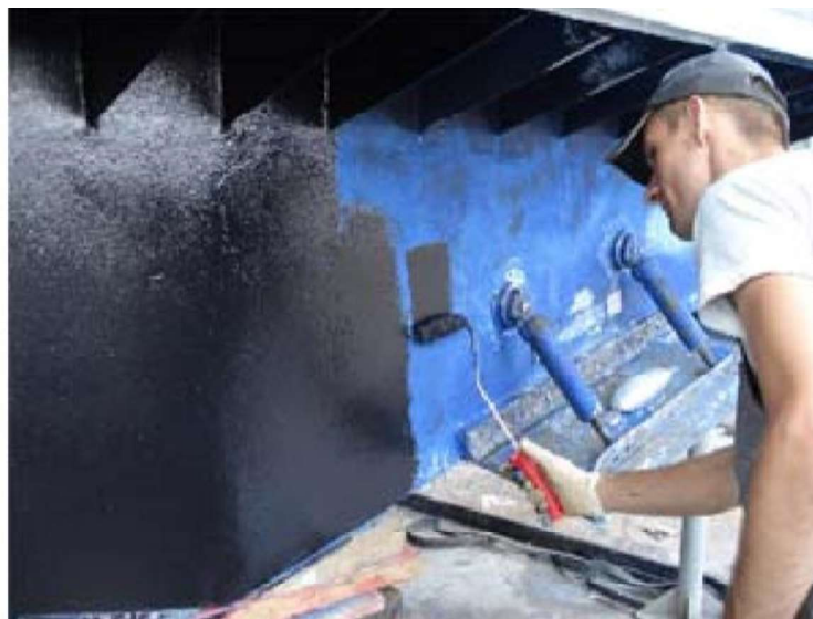
Figure 4. Application by roller
