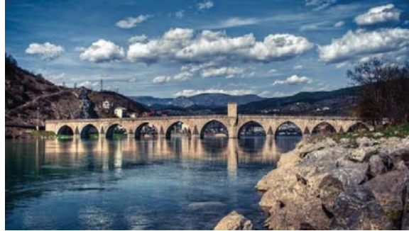
b) Stone road pedestrian bridge [6]
