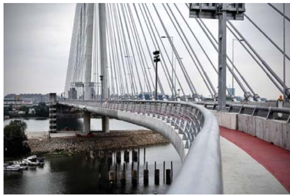
d) Road railway pedestrian bicycle reinforced prestressed concrete bridge with steel ropes [8]
