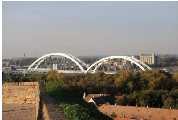
c) Road railway metal concrete bridge [7]
